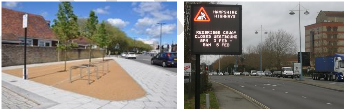
Platform Road improvements (left) and new Enhanced Variable Message Signs
